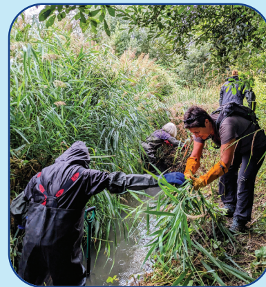
Clearing the river channel
